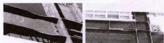
Figure 2. Application of Reduced Beam Section (RBS) Connection
