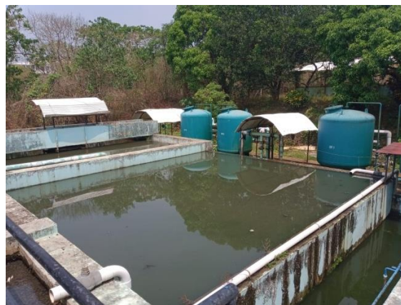
Fig. 3.2 d: Secondary Clarifier
