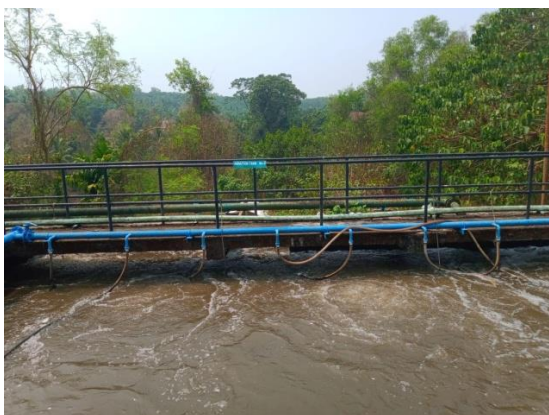
Fig. 3.2 c: Aeration tank
