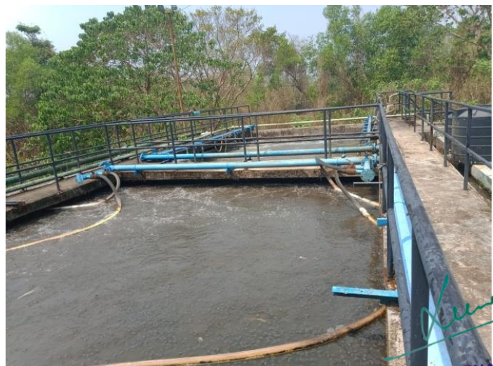
Fig. 3.3 b: Aeration tank
