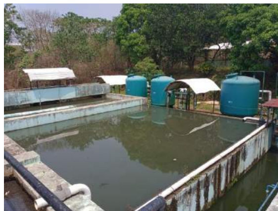
Fig. 3.2 d: Secondary Clarifier
