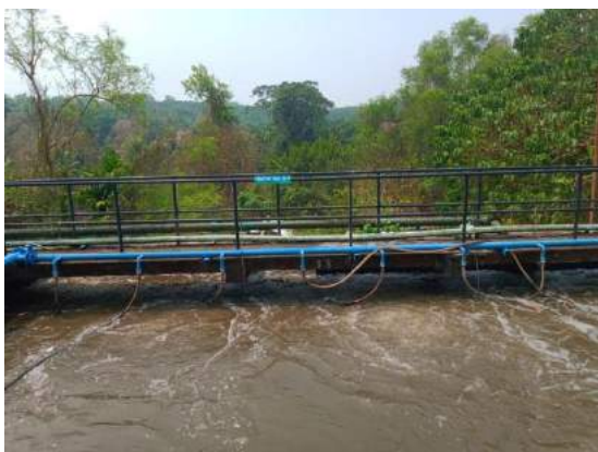
Fig. 3.2 c: Aeration tank
