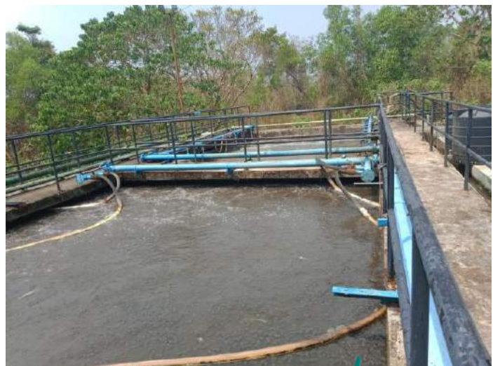
Fig. 3.3 b: Aeration tank
