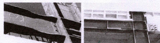
Figure 2. Application of Reduced Beam Section (RBS) Connection
